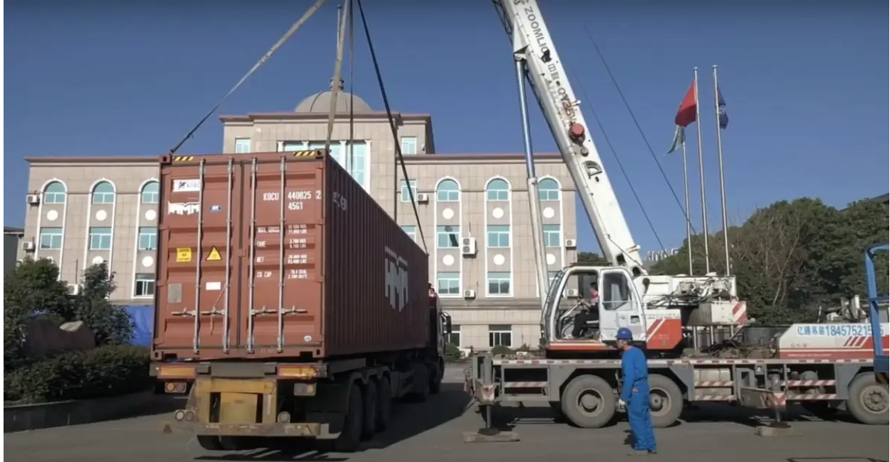
The folded unit being lifted by the crane. Hapi Homes/YouTube
