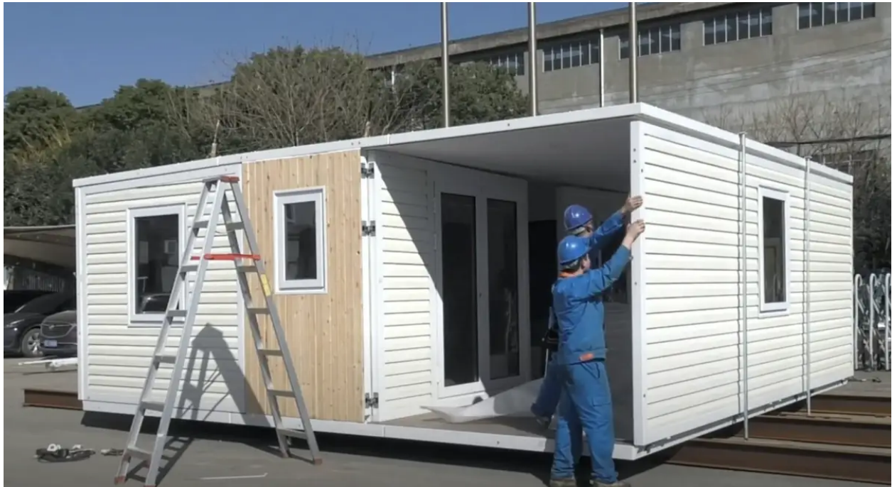
Builders towards the end of unfolding the exterior walls. Hapi Homes/YouTube
